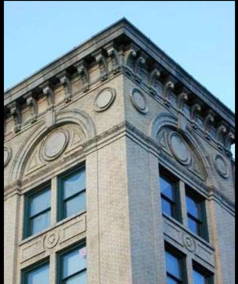
Holley Mason Building, Spokane
