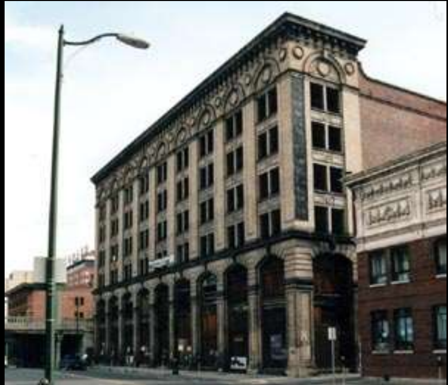
Holley Mason Building, Spokane
