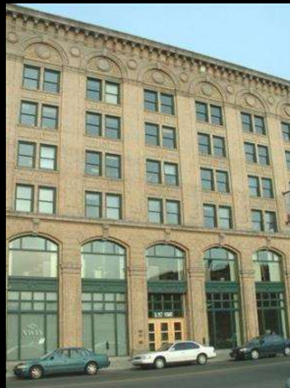
Holley Mason Building, Spokane
