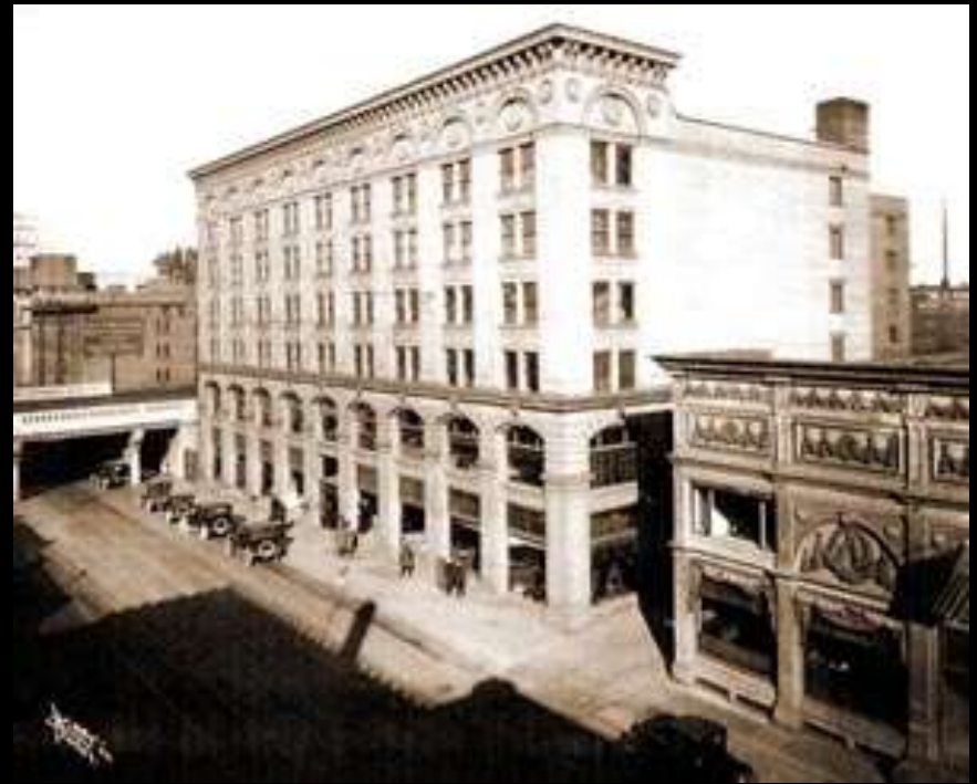
Holley Mason Building, Spokane
